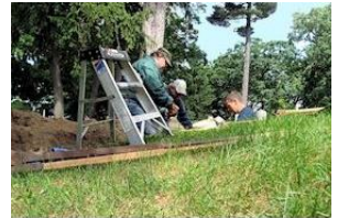
Brothers digging the hole for the foundation.
