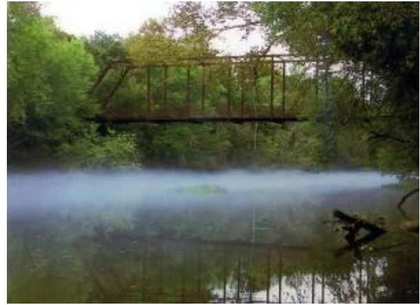
The bridge over the Green River at Tebbs Bend, KY. The iron bridge was rebuilt on the original stone pilings in 1907 to replace the wooden covered bridge built in 1863.
